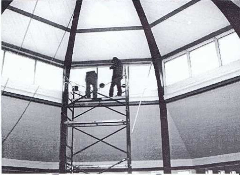
The present Chapel being re-roofed, re-painted and re-clerestory windowed
