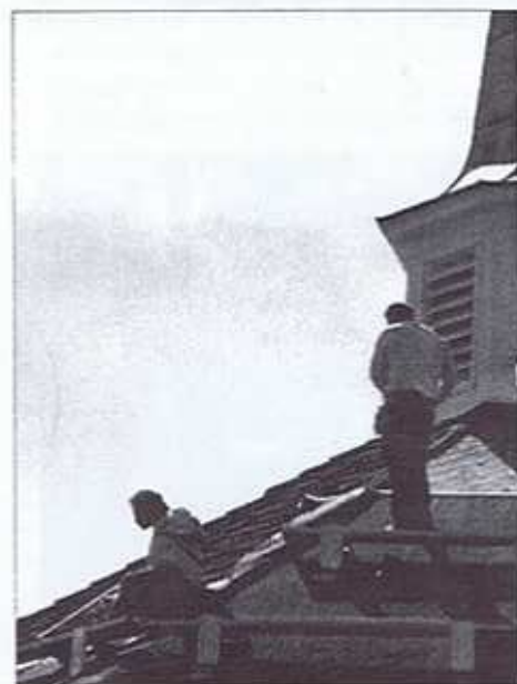
The roof and steeple in process...
